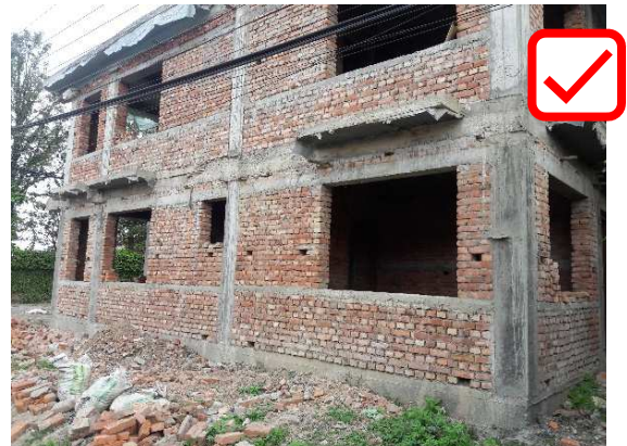
Wall braced by horizontal band
