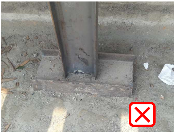
Simply rested on the ground
