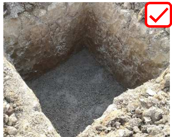
Well compacted earth
