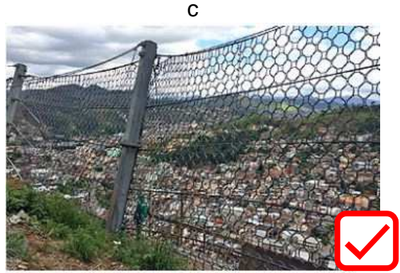
Rockfall protection work
