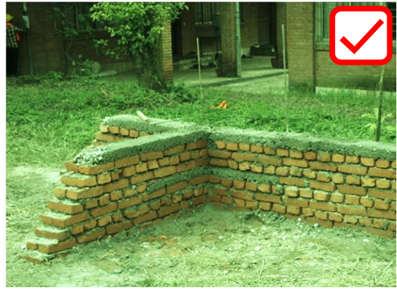
Stepping left for later construction joint
