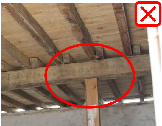
Post simply supporting floor
