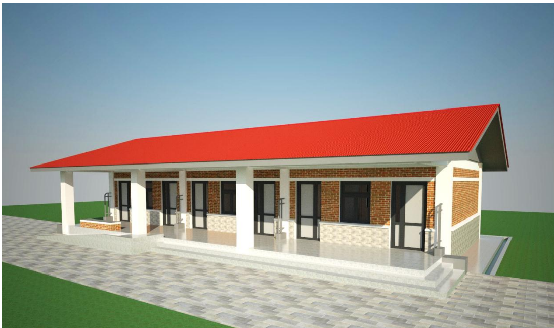
Practical Block, 1 Storey
