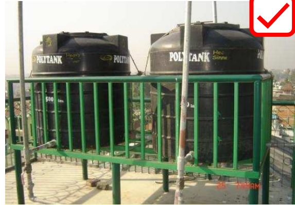
Safe placing of water tanks
