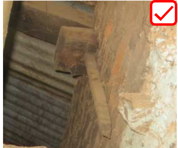
Wooden member laterally restrained
