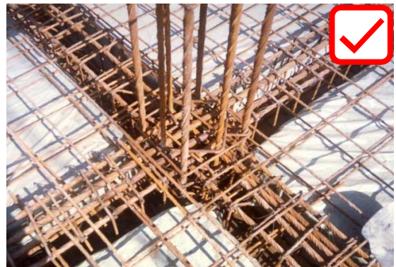
reinforcements of beam confined by column reinforceds
