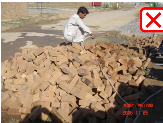
Just spraying water over brick before laying
