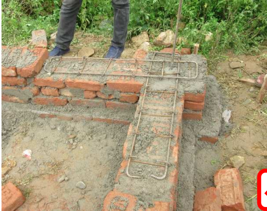
Reinforcement placing for stitch bands
