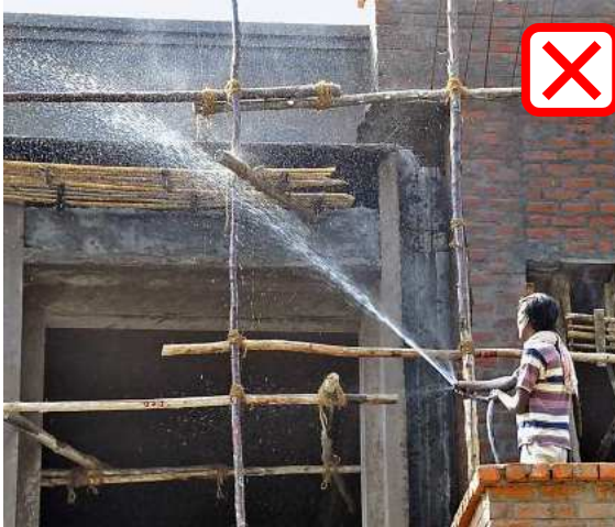
Curing with water sprinkling only
