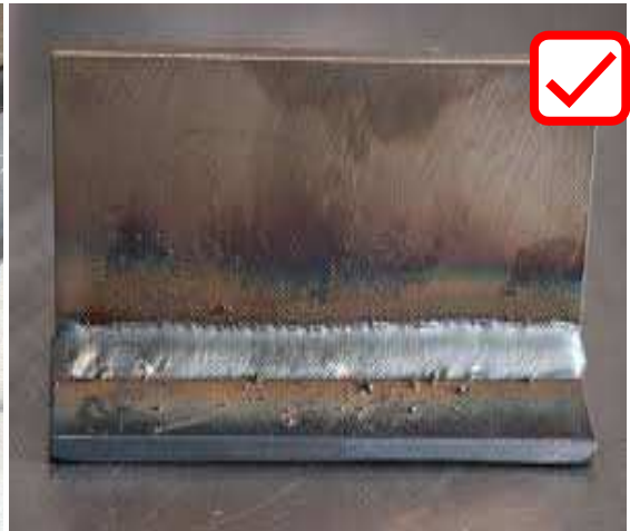
Proper through welding
