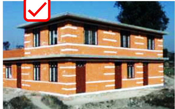
Masonry wall with bands and vertical reinforcement.
