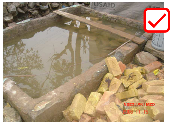
Bricks immersed in water before laying
