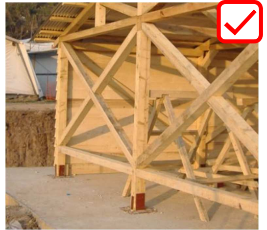
Proper Wooden connection at ground floor level
