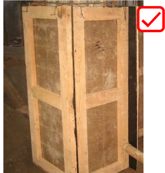
Proper method of formwork
