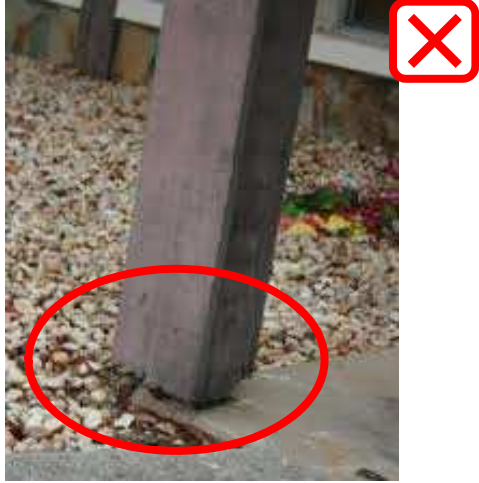
Wood without protection at ground
