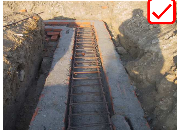
Foundation band in masonry structure
