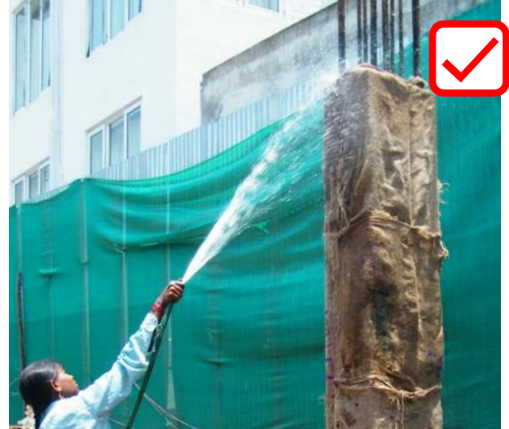
Curing with Jute sack
