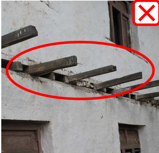
Wooden member simply resting on floor
