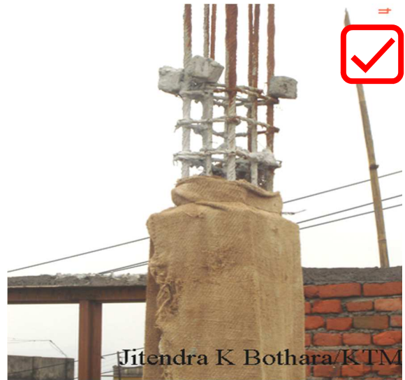
Proper use of Cover block
