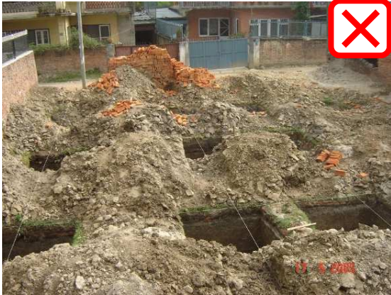
Excavated soil cleared from site
