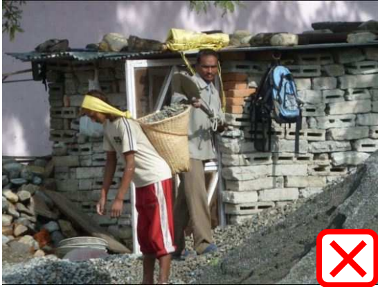
Measurement of ingredients by unstandard container
