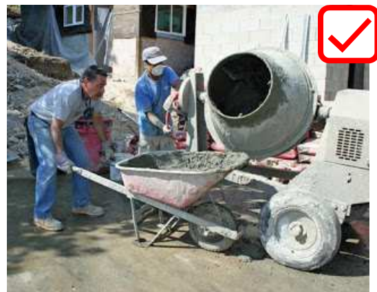
Concrete mixing by machine
