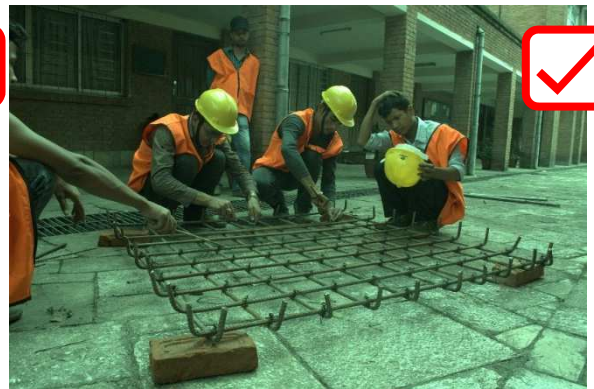
Ends of the footing mesh bent up
