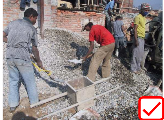
Measurement of ingredients by standard box
