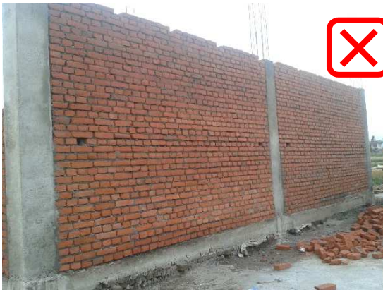
Wall without horizontal band
