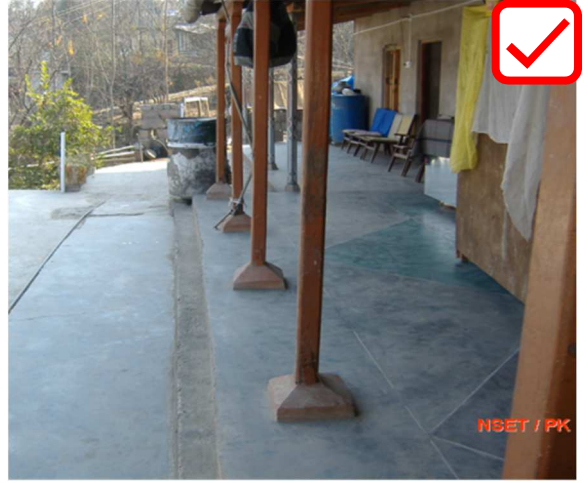
Wood protected at its base
