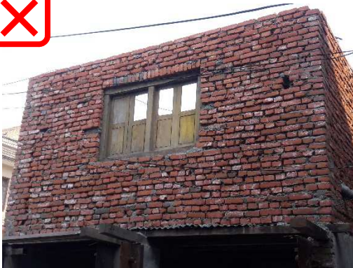
Masonry wall without bands
