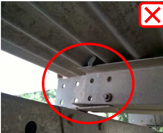
Weak joint with single nut bolt
