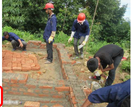
Reinforcement placing for stitch bands
