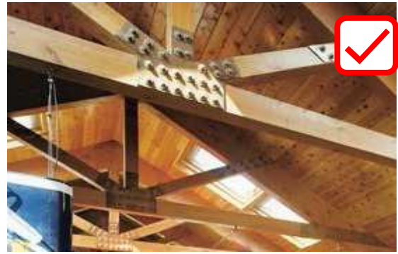
Proper connection of members of wooden truss
