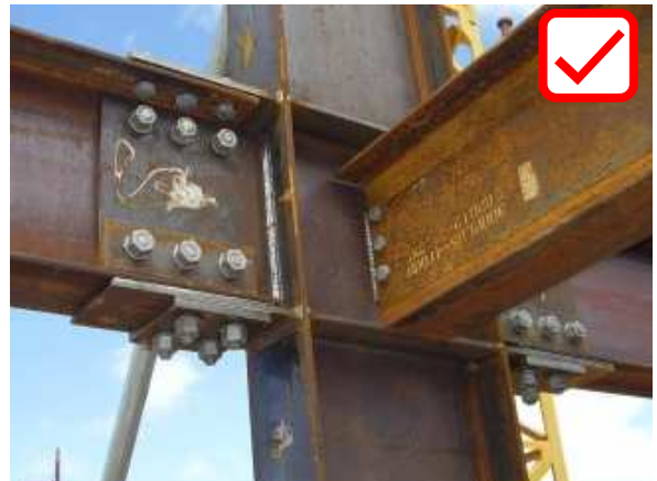
Proper connection as designed
